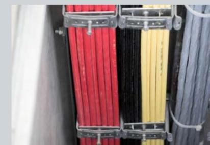
Triax, video and audio cables made by Draka Communications - extreme space ratio and still optimal transmission characteristics.
